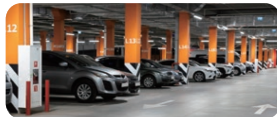
Smart Parking Lot
